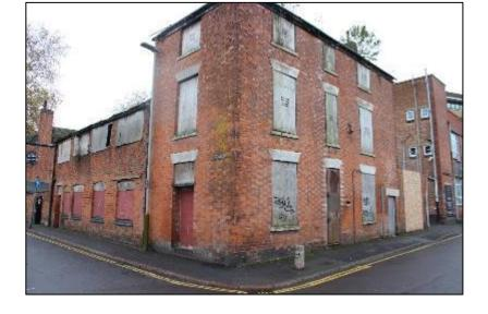
The building is in immediate risk of further deterioration, suffering from long-term vacancy and lack of maintenance. The former workshop is structurally unstable, whilst the main structure displays substantial failure of roof cover and structural cracking to brickwork. The site also suffers from unauthorised access, vandalism and pigeon infestation.
