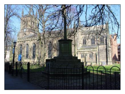
The church remains occupied and in fair condition, suffering from localised decay and issues immediately related to the churchyard, with overgrown vegetation blocking the guttering and damage caused by vandalism & anti-social activity.
