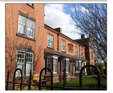
The property is suffering from progressing deterioration and lack of regular maintenance. Of most concern are the deteriorated original sash windows, with one unit missing.
