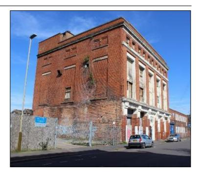
The building is in slow decay, suffering from long-term unoccupancy, minor fire damage and failing rooflights.
