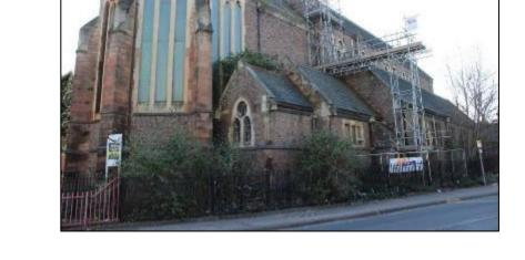
The former church remains vacant and in immediate risk of further deterioration. It has a failing roof covering, allowing water ingress into the building, causing damage to internal surfaces and architectural features.
